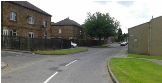
Figure 11. Road Access to Hendon Court
